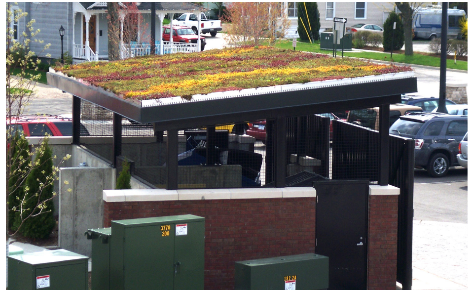
Green roof over trash/recycling enclosures in Grand Haven.
